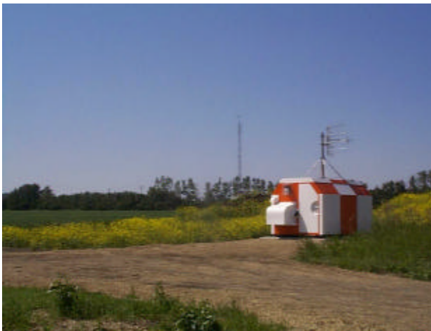
Figure 4: Ground Entry Station at Edmonton
